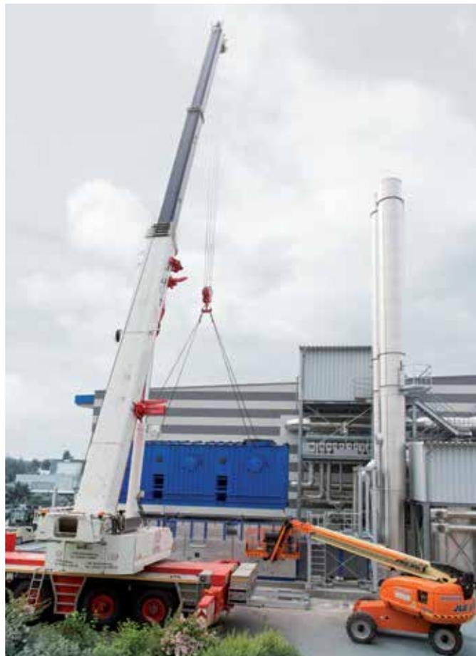
Figure 2: An *Ecopure*® RTO plant from Dürr is being erected.
